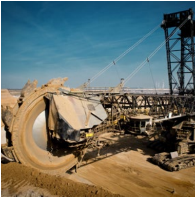
Bucket wheel excavators
